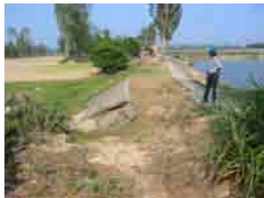
Few of the many easily damaged sections of the salinity dyke system along Tra Bong River (Quang Ngai).
