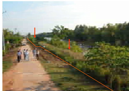
... and along the edge of flood resettlement centers. The red line shows about 5 m of dry land is saved thanks to Vetiver grass.
