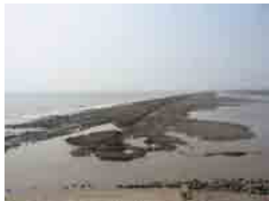
A very rigorously built sea dyke in Hai Hau (Nam Dinh) ... and what is left from the previous dyke, about 200 m sea-ward and built 20 years ago.
