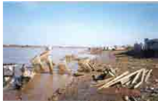
Bank erosion along Ganh Hao River (Bac Lieu), causing complete collapse of the jetty.
