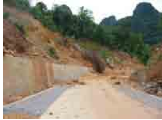
Even concrete retaining wall did not help - a rock slide near Phong Nha (Quang Binh).
