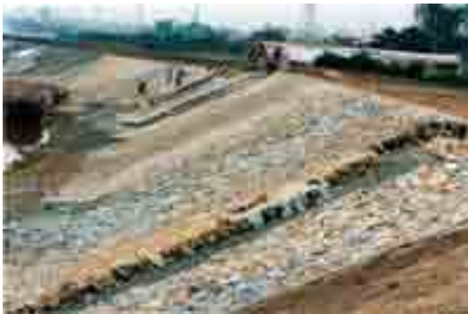
A rigorous rock riprap dyke along the Red River in Hanoi ... And washed into the river.
