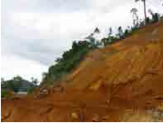
Landslide in the completely weathered granite along Ho Chi Minh Highway (Thua Thien-Hue).
