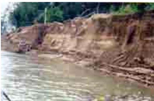
Right bank erosion along Tra Khuc River in Quang Ngai.
