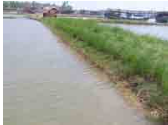
... On both sides of an anti-salinity estuary dyke along the same river.
