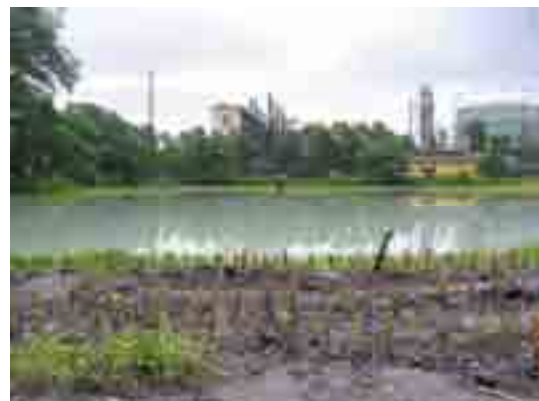
An environmental pond at the fertilizer plant in Bac Giang province which can't help reducing suspended/soluble toxic elements.
