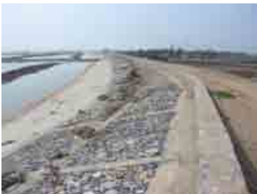
A very rigorously built sea dyke in Hai Hau (Nam Dinh) ... and what is left from the previous dyke, about 200 m sea-ward and built 20 years ago.
