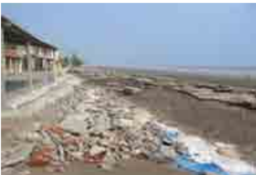
Coastal erosion in Hai Hau (Nam Dinh) due to storm No. 7 - a used to be nice walkway.
