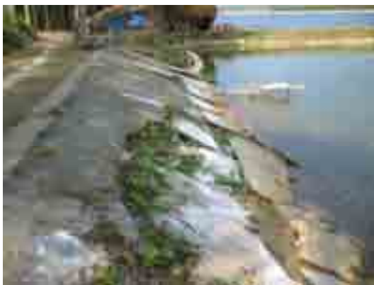
Few of the many easily damaged sections of the salinity dyke system along Tra Bong River (Quang Ngai).
