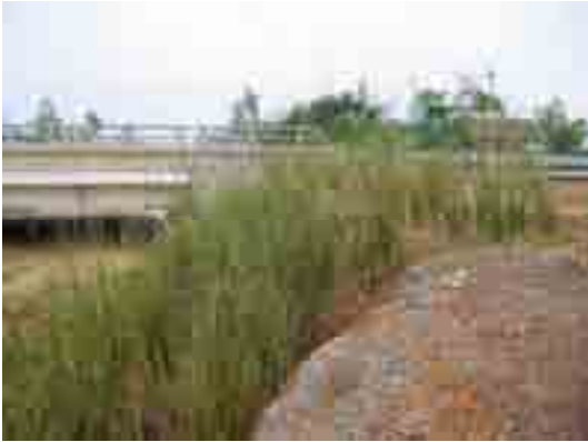
Vetiver grass for protection of bridge abutment along the No. 1 National Highway.
